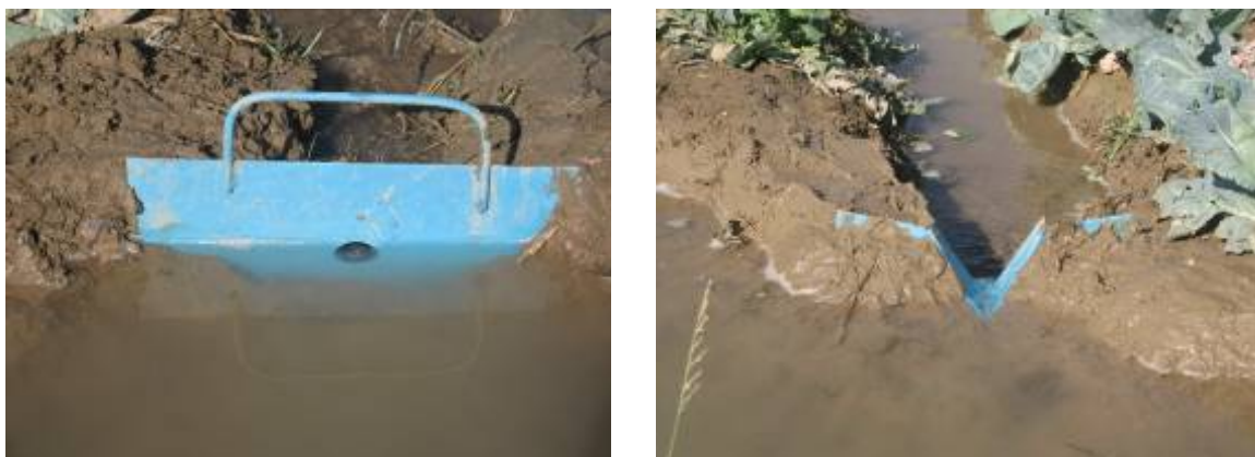
Figure 1 - Watering shields for the measurement of water flow in the furrow
